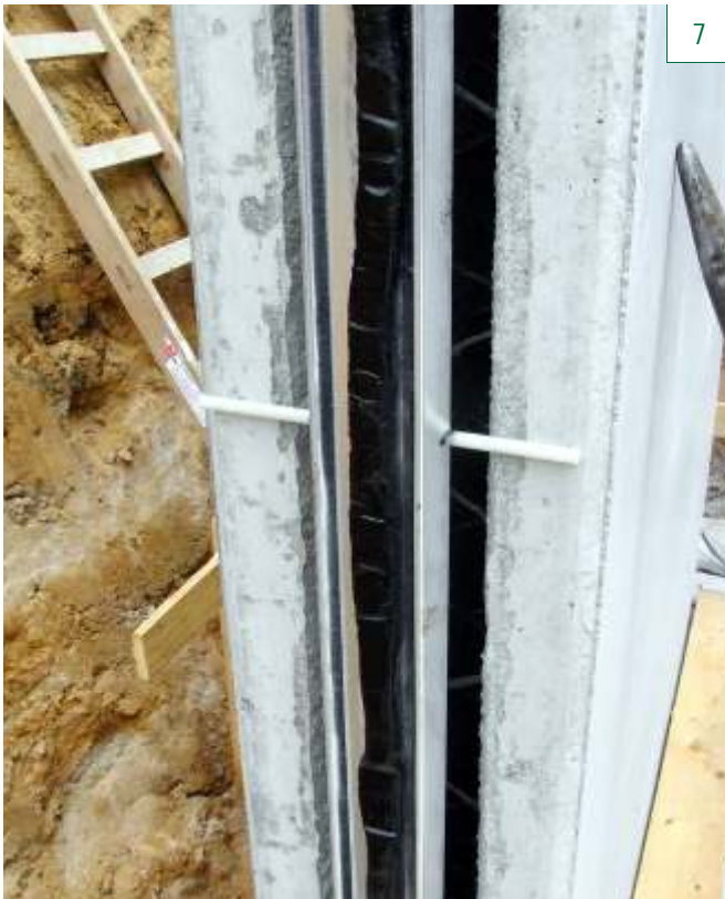
Crack inducer in a prefabricated wall butt-joint
