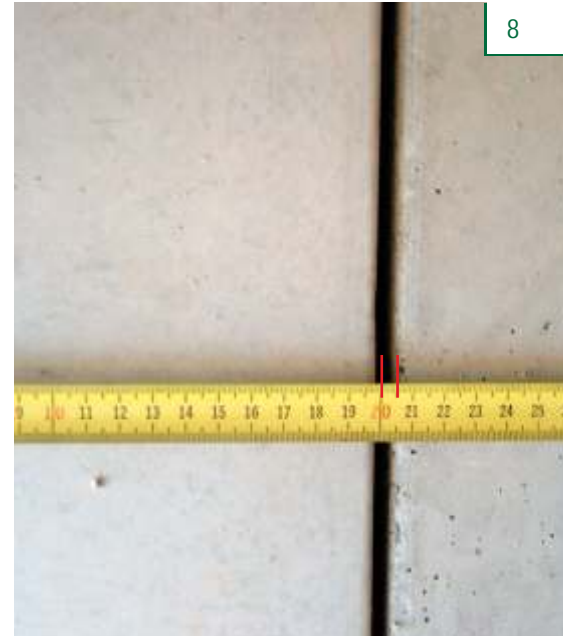
Final joint thickness about 5mm
