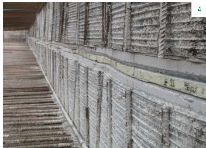
Working joint of two bottom slabs
