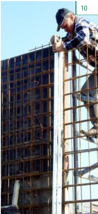
Crack inducer in an in-situ concrete wall
