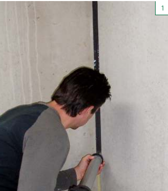
InnoElast® as joint finishing
