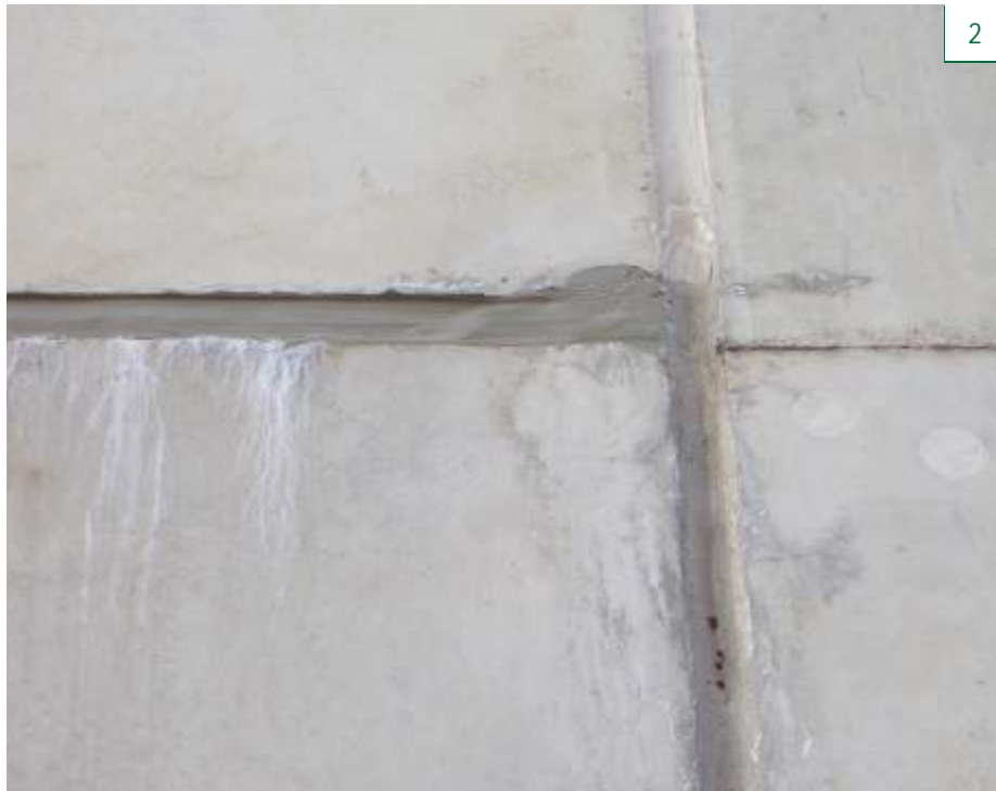
InnoElast® for joint repairing
