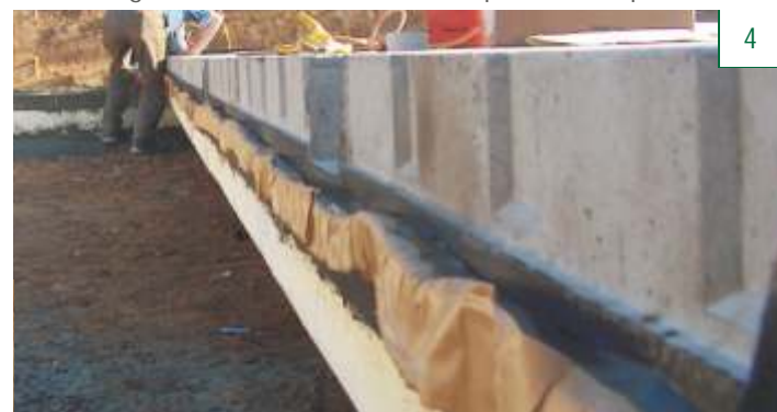
Sealing between bottom slab components
