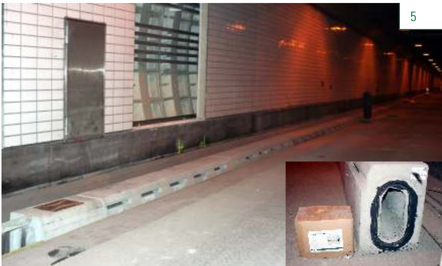
Firm gluing of pre-cast components
