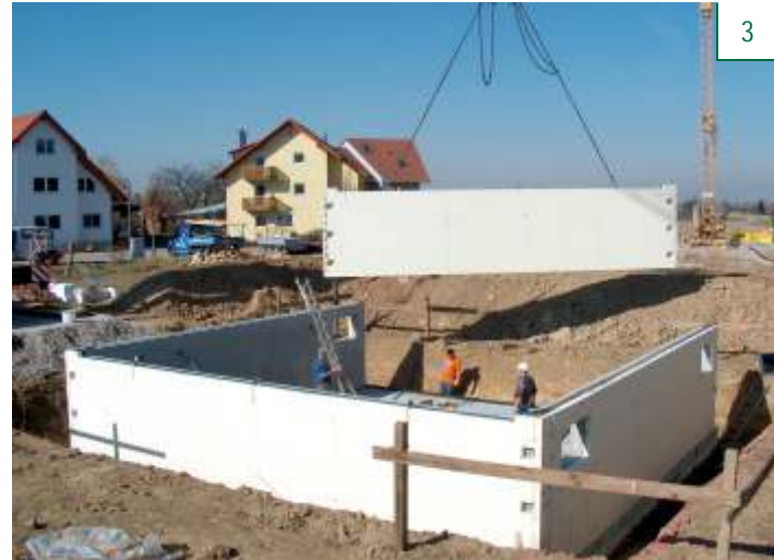
Watertight basement made of massive pre-cast components
