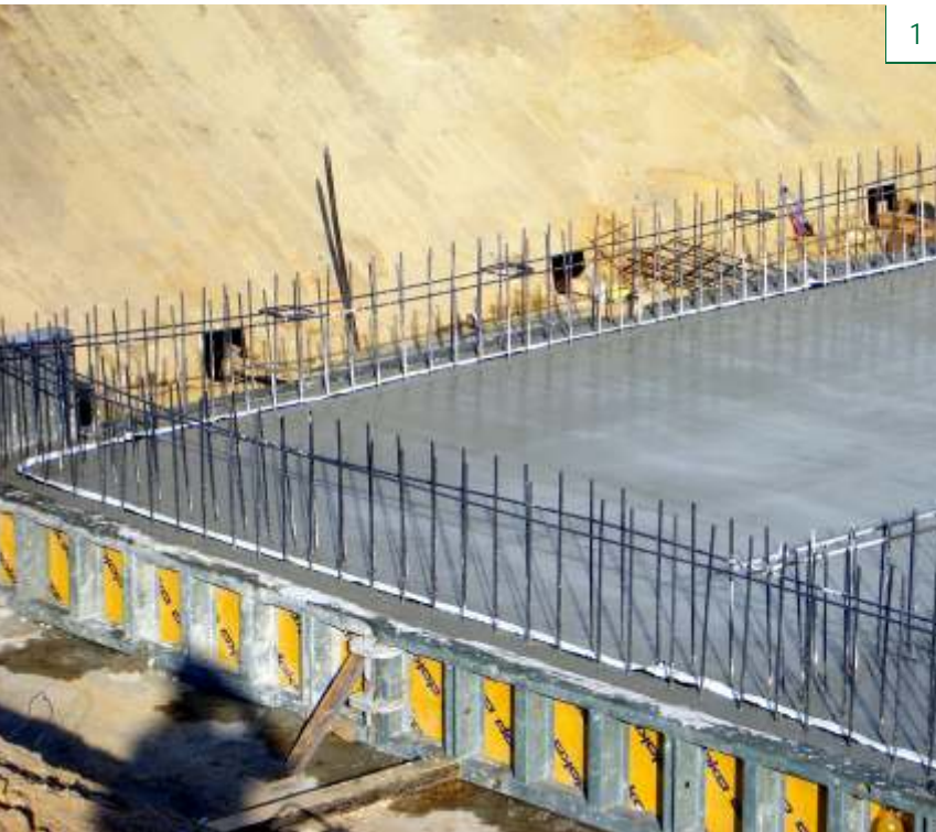
Working joint of a bottom slab and a wall
