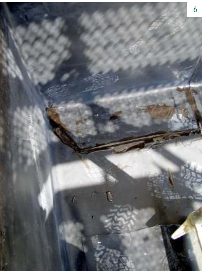
InnoElast® as a glue for EPDM films
