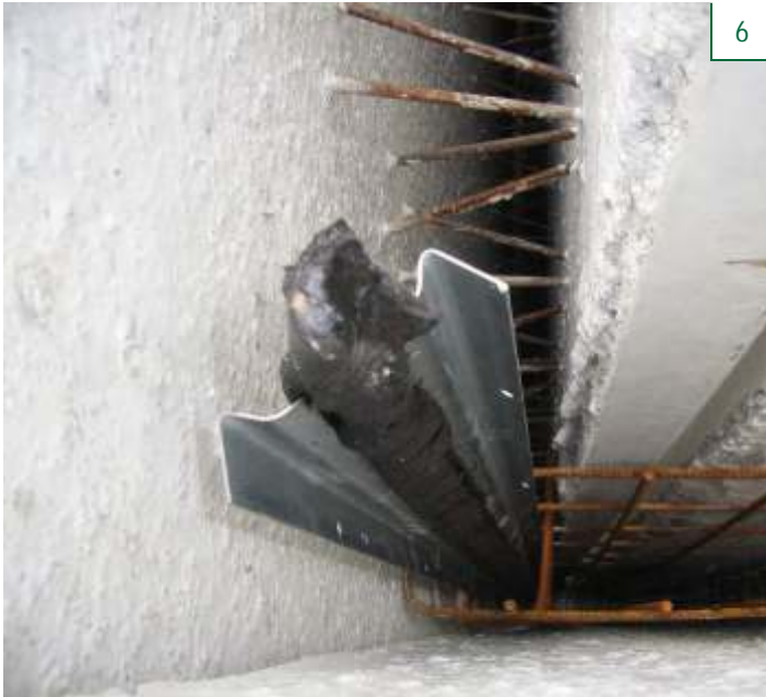
Crack inducer in a prefabricated wall/ceiling with reinforcement
