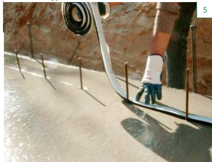
Placing in fresh concrete
