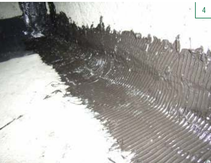
InnoElast® as “liquid foil”
