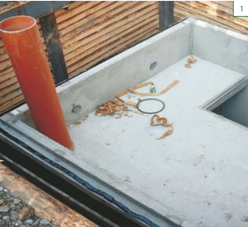
Sealing of shaft joints
