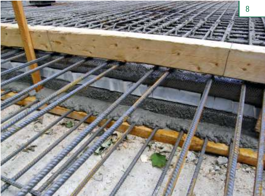
Shuttering element in the bottom slab
