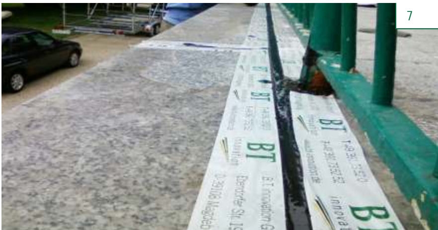
InnoElast® as sealing for floor joints
